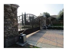
This component is for the replacement of the decorative metal vehicle gates along Fowler Avenue. The gates and hinges appeared to be in good condition without any sign of damage or rust. With proper maintenance, the useful life could be greatly extended. Painting is provided for within another component.
