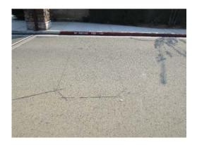
This is for the replacement of the underground sensor loops and the pulling of new wire harnesses. The current harnesses were functioning properly at time of inspection. If possible, loop replacement should be scheduled to coincide with paving repairs or gate operator replacement.
