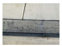
This component covers the maintenance and repair of the curb and gutter throughout the development. The curb and gutter appeared to be in fair condition with some areas of chipping and cracking. This component should last the life of the development with proper maintenance. Such maintenance may include crack fill, grinding, efflorescence removal, sealing, etc. We estimate 2% will require repair every 5 years.
