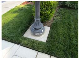
This component covers the painting of the street light posts. There are areas of noticeable wear. Painting is used to prolong the remaining life of metals because this can prevent rust and corrosion. The painting preparation should include power washing, scraping and repair if needed.
