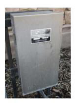
The lighting is controlled by a Vista model MT1200 power transformer. This item appeared to be in fair condition. The functionality was not observed. This component is for the replacement and reinstallation of the item.
