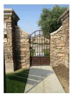
This component is for the replacement of the metal pedestrian gates. The gates appeared to be in good condition without any sign of damage or rust. With proper maintenance, the useful life could be greatly extended. Painting is provided for within another component.
