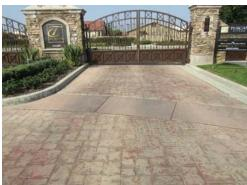
The stamped concrete paving at the entrance of the development appeared to be in fair condition with cracking noted throughout. The life of this component will exceed the scope of this 30 year study. This component should last the life of the development with proper maintenance. Periodic maintenance may include mechanical and/or chemical cleaning, efflorescence removal, sealing, grinding, etc. We estimate 5% of the concrete will require repairs every 5 years.
