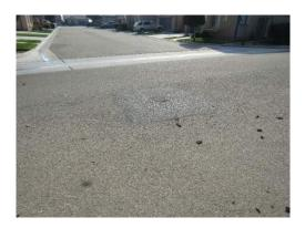
There is approximately 319' of concrete valley gutter in the development. The component is for the repair and replacement. The current condition of the concrete was good. Periodic maintenance may include efflorescence removal, sealing, grinding, crack fill, or replacement. We estimate 5% will require repair every 5 years.
