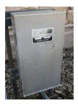
The lighting is controlled by a Vista model MT1200 power transformer. This item appeared to be in fair condition. The functionality was not observed. This component is for the replacement and reinstallation of the item.
