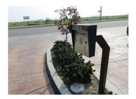
The entry keypad is a DoorKing DKS model 1834. It appeared to be in fair condition without any sign of damage or malfunction. Typically, if the keys show signs of wear or sticking, the key code can be changed to less frequently used numbers to extend the life of the component and provide more equal wear.
