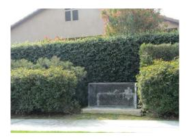
This component covers the replacement of the backflow preventers. They appear to be in fair condition, enclosed in metal mesh crates.
