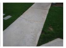
This component involves the ongoing maintenance and repairs of the concrete pavement located throughout the common areas of the development. Annual inspections are essential to identify and correct any elevation changes or trip hazards for which the association could be held responsible. If cracks are not addressed promptly, moisture can penetrate and cause further deterioration. Overall, the concrete is in good condition, with no visible cracks present.
