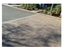
The stamped concrete paving at the entrance/exit of the development appeared to be in fair condition with cracking noted throughout. The life of this component will exceed the scope of this 30 year study. This component should last the life of the development with proper maintenance. Periodic maintenance may include mechanical and/or chemical cleaning, efflorescence removal, sealing, grinding, etc. We estimate 5% of the concrete will require repairs every 7 years.
