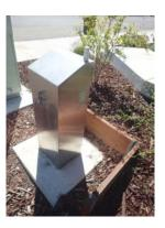
This component is for the replacement of the irrigation controllers. The controller appeared to be in good condition with no signs of operational problems. Irrigation controllers usually have a normal useful life ranging from 8 to 15 years depending on the unit type and the
