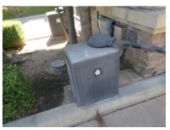
This component is for the replacement of the gate motor/operators servicing the main entrance/exit gates. The function of the operators was observed and noted to be functioning properly without any sign of defect. Regular maintenance is recommended to prevent premature failure and further help prolong its useful life.
