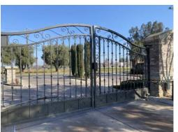
This component is to prepare, power wash, sand, scrape, spot prime, and paint the wrought iron gates and fencing. To ensure the wrought iron achieves its full useful life, it should be painted as recommended. The paint on the gates was in overall fair condition. Without proper paint maintenance, the useful life of wrought iron can be greatly diminished.
