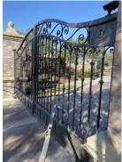
This component is to replace the decorative metal vehicle gates. The gates and hinges were in good condition, showing no signs of damage or rust. With proper maintenance, their lifespan could be significantly extended. Painting is included under a separate component.
