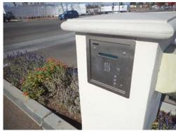
The entry keypad is a DoorKing model 1830 and appeared to be in good condition with no visible damage or malfunctions during the inspection. If the keys begin to show wear or become sticky, the key code can be modified to include less frequently used numbers, helping to extend the component's lifespan and distribute wear more evenly.
