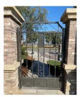
This component is for the replacement of the metal pedestrian gates. The gates were observed to be in good condition, showing no signs of damage or rust. With proper maintenance, their lifespan could be significantly extended. Painting is included as part of a separate component.
