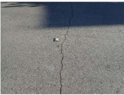
This component involves the preparation of asphalt and the application of a slurry seal coat. A seal coat is a thin liquid layer that acts as a sealant, helping to protect against damage from environmental factors. This component comprises striping, crack filling, skin patching, minor excavation and backfill, etc. If an additional coat is desired, the overall cost typically increases by 10% to 20%. Cracks that are 1/4" or wider should be filled once detected. The observed condition was fair.
