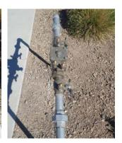
This component covers the replacement of the backflow preventers. They appeared to be in fair condition at the time of inspection. We recommend having them covered by an insulated pouch to help prevent corrosion and further extend its useful life.
