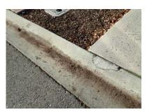
This component covers the maintenance and repair of the curb and gutter throughout the development. The curb and gutter appeared to be in fair to poor condition with some areas of chipping and cracking. This component should last the life of the development with proper
